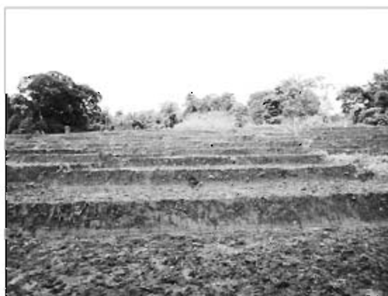
Bench Terrace at Snal Dajreng under Manda Watershed, IWMP-I
