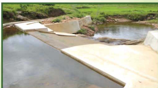
RCC Diversion Dam At Mukhla
