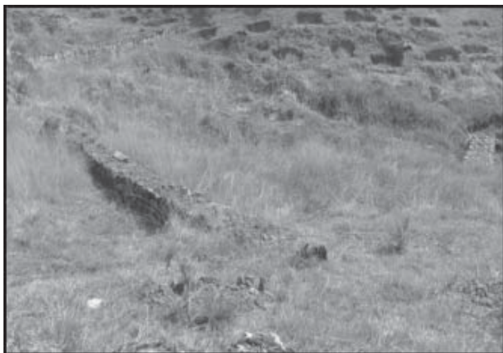
Loose Boulder bunds to minimise erosion and facilitate infiltration
