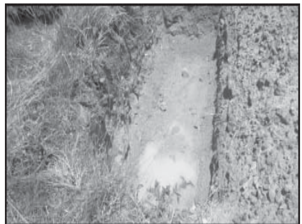
Contour Trench For Spring Recharge
