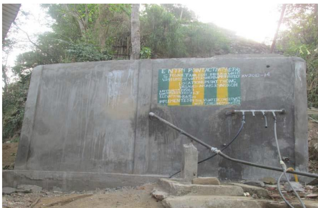
SPRING TAPPED CHAMBER WATER CUM WATER STORAGE TANK
