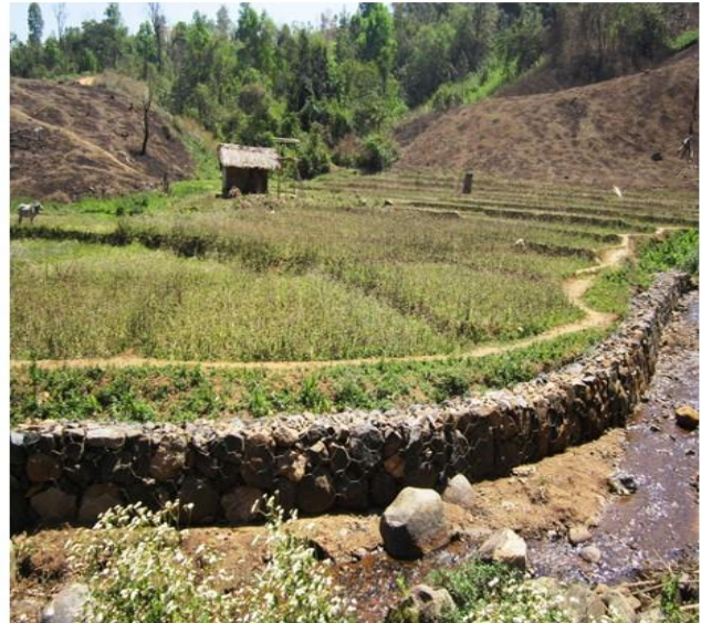
Boulder Sausage Protection wall at Rongal Watershed, East Garo Hills IWMP-II
