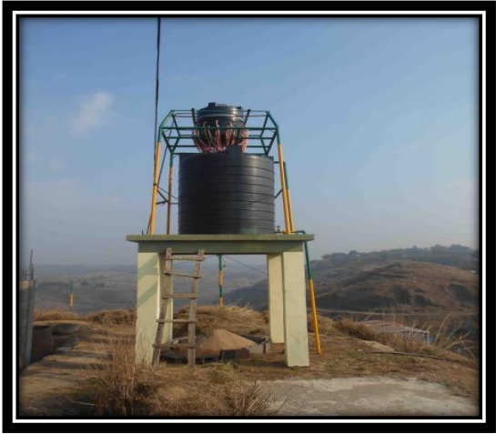
Overhead tank for filtering, storing and distributing potable water
