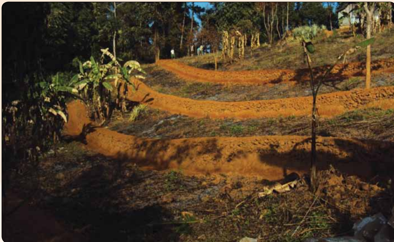
Activity- Countour Bunding, Batch-II (IWMP-IV) | Watershed - Lower Umpih Watershed Village- Mawtari Myrdon | C&Rd Block-Umsning | District- Ri Bhoi
