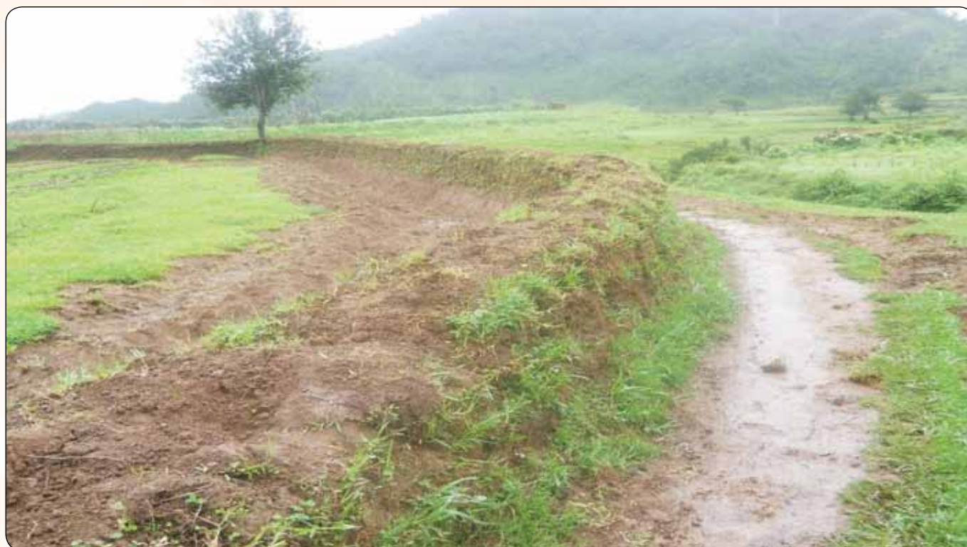
Peripheral Bunding Under Wah Umlingdoh IWMP IX, East Khasi Hills
