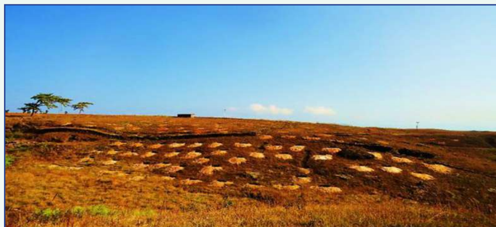
Activity: Staggered Contour Trenches
