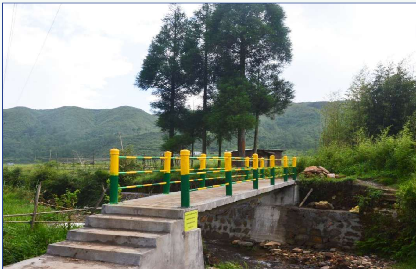
Foot Bridge Structure (Infrastructure Development) under Wah Lyngkien Phase-I RIDF-XXIV, Ramklang, East Khasi Hills
