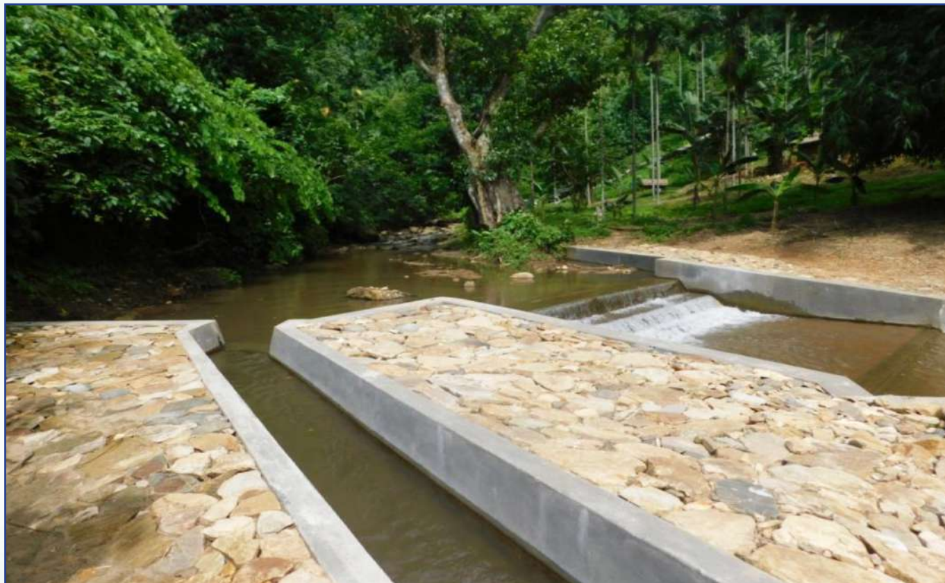
RCC Irrigation Dam with Channel under Middle Chill AIBP Project, North Garo Hills
