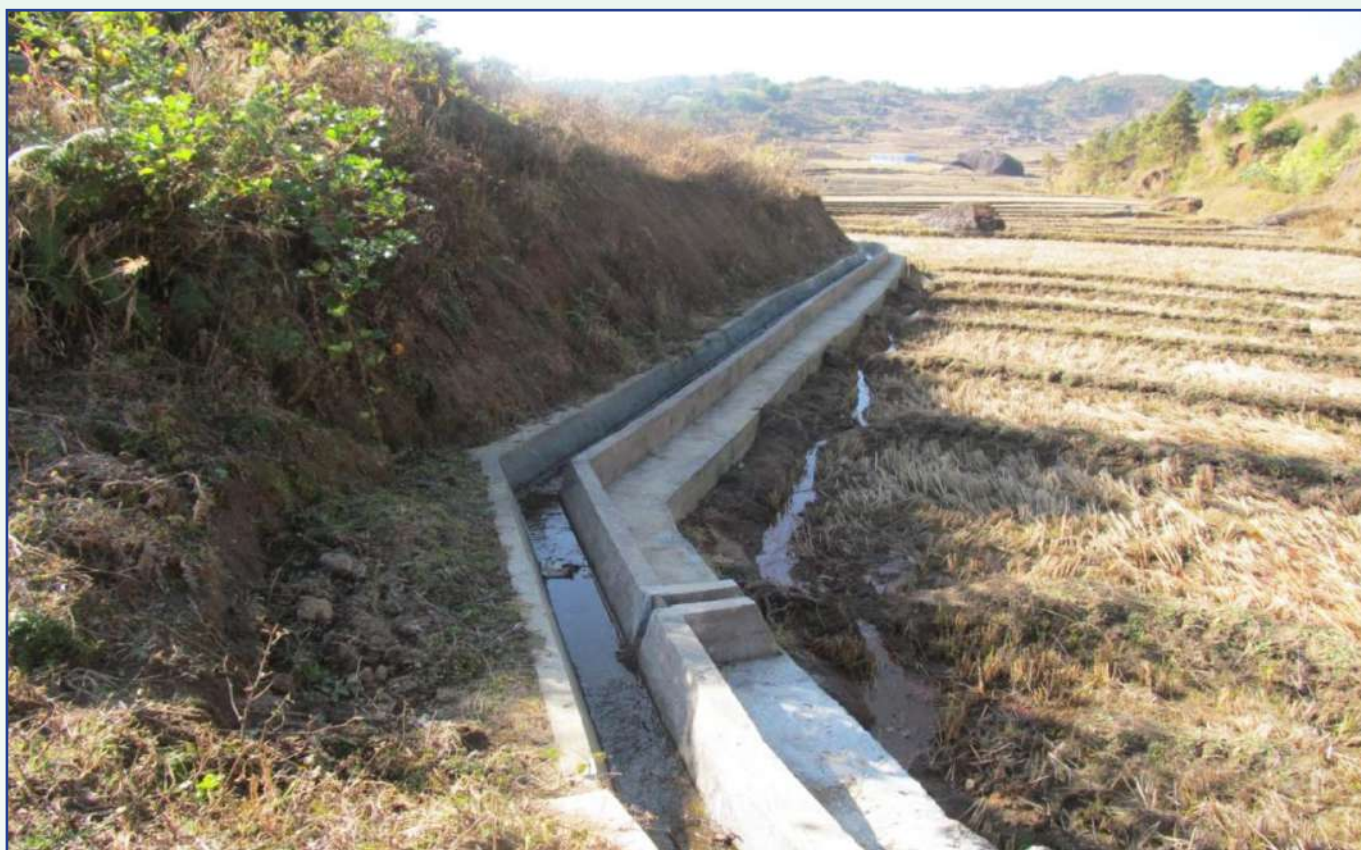
CC Channel Structure under Wah Tyrkhang AIBP Project, South West Khasi Hills
