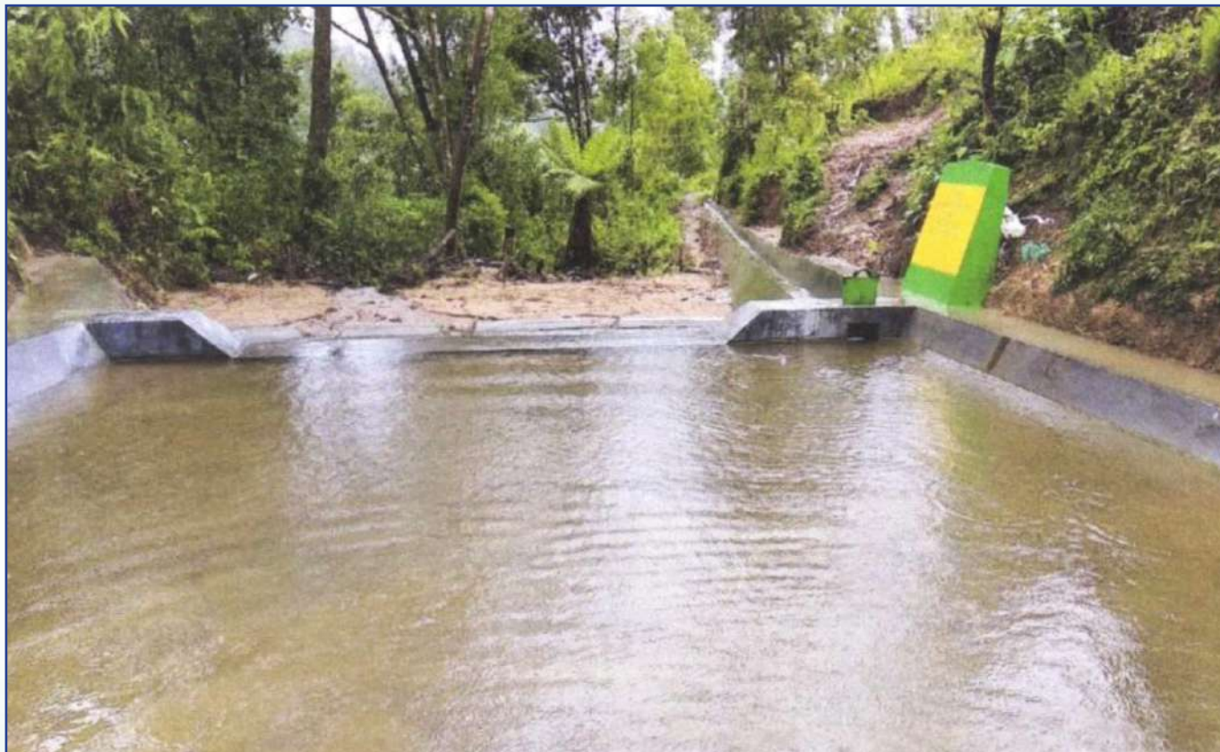
Diversion Structure under Wah Lalip RKVY, Shangpung Moosiyem, West Jaintia Hills
