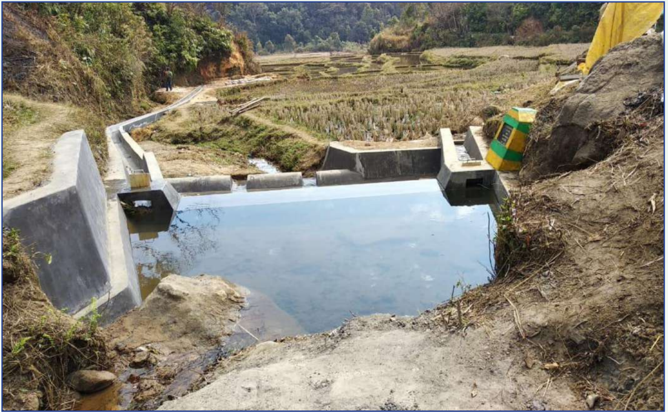
RCC Dam and Channel under Ramut-Umpaai RIDF-XXIV, Wah Lynger, West Jaintia Hills
