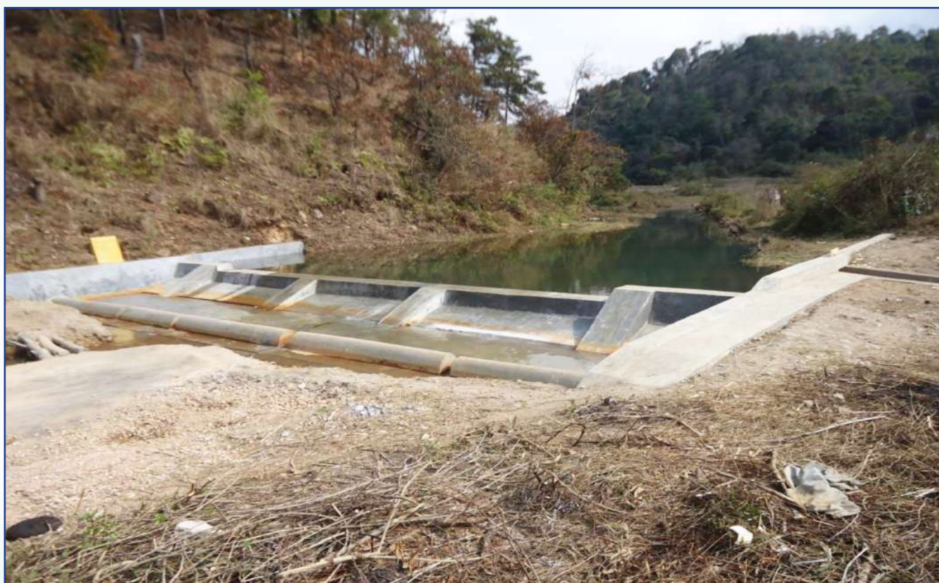
CC Dam under Nongjingi AIBP Project, West Jaintia Hills
