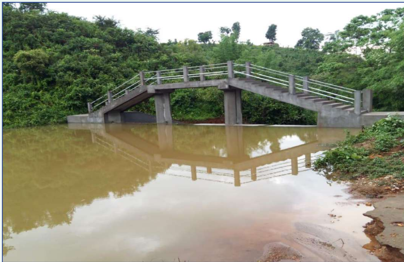
Water Harvesting Structure under Lower Sugri RIDF-XXIV, Balupara, West Garo Hills
