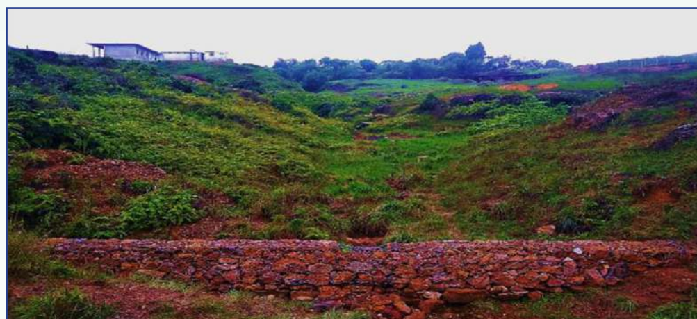
Activity: Loose Boulder/ Gabion Check Dam
