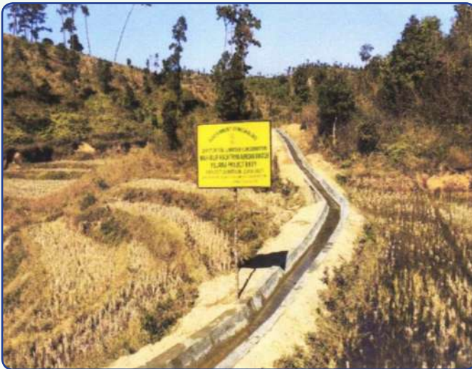
Conveyance Structure No. 1
