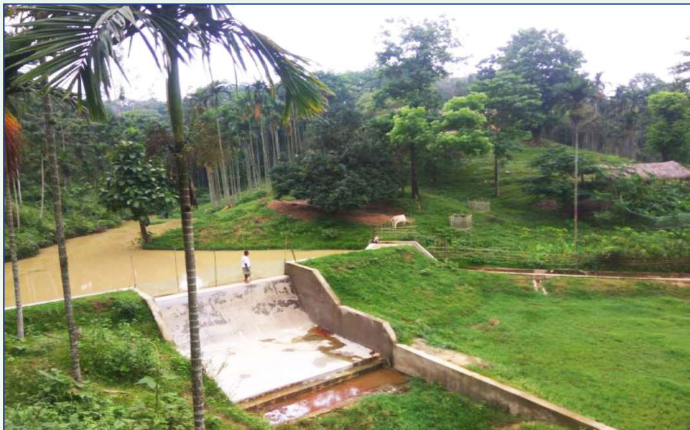
RCC Irrigation Dam & Channel under Balda RVP, South Garo Hills
