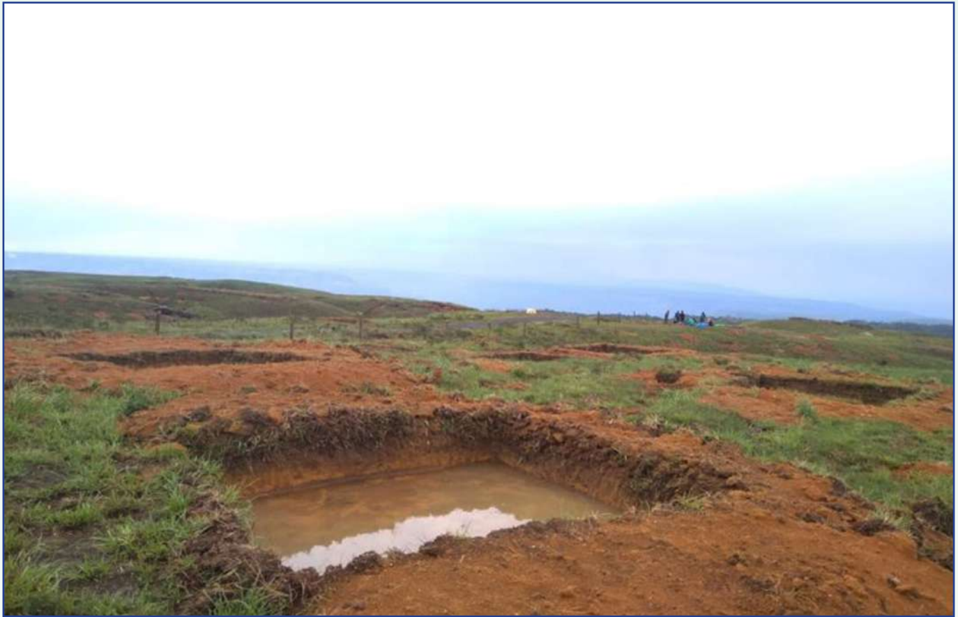
Percolation Pits in Recharge Area
