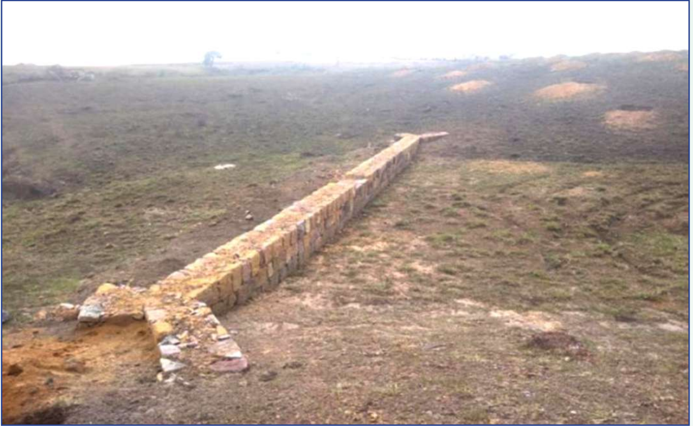
Loose Boulder Dam to trap runoff and facilitate infiltration
