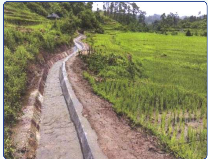
Conveyance Structure No. 2
