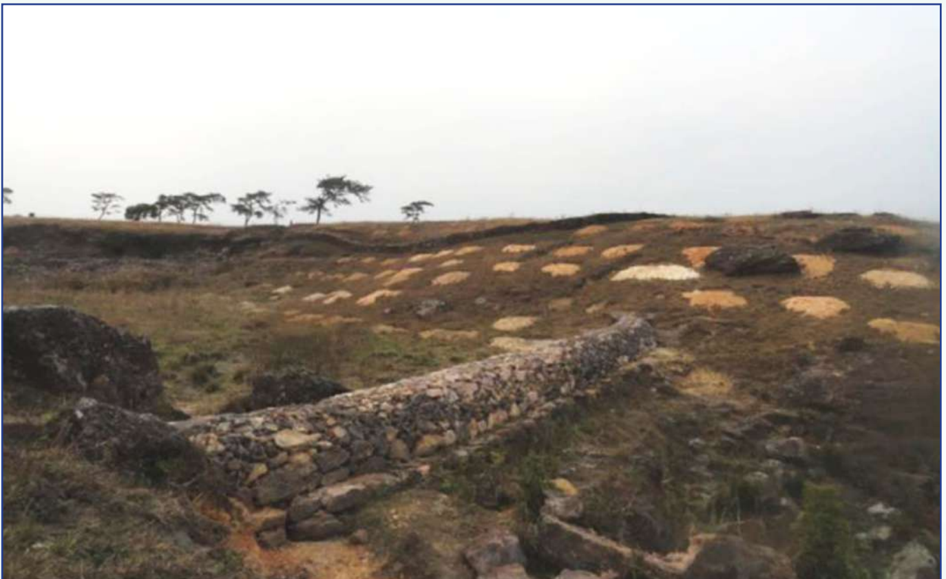
Loose Boulder Dam with trenches
