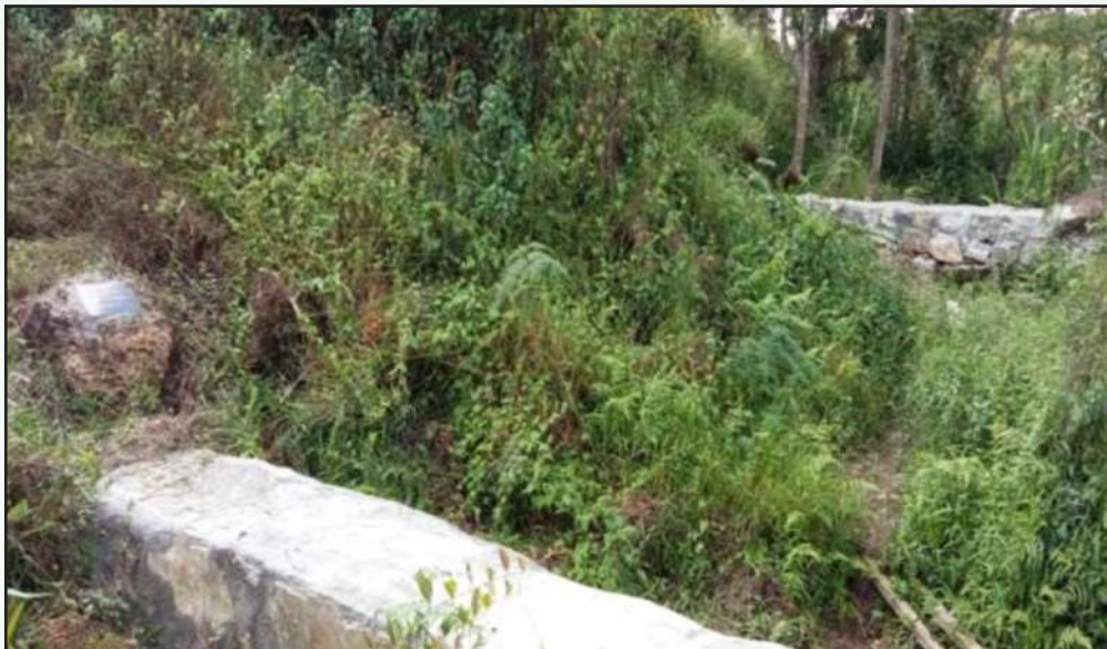
Activity: Check Dam Village: longkaluh
