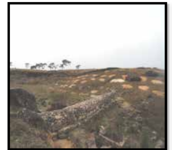
Loose Boulder Check Dam
