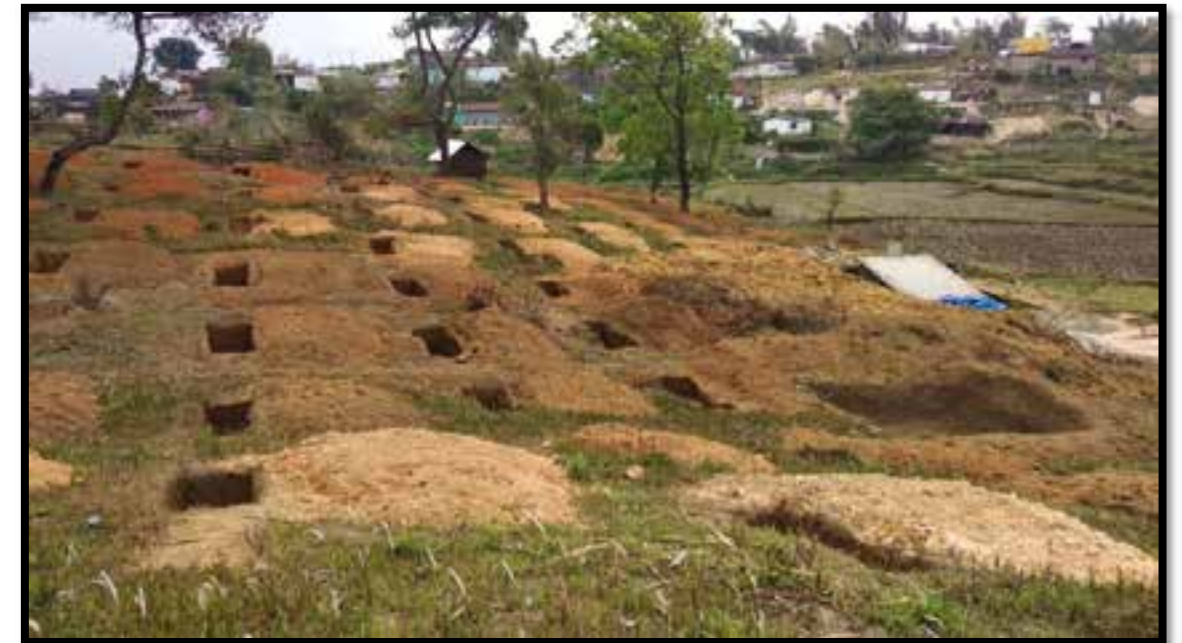
Trenching works in the Springshed Recharge Areas
