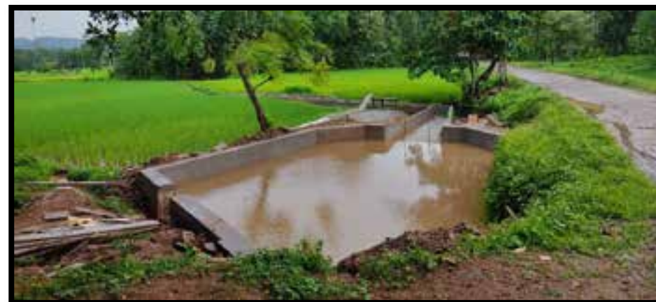
Protection Wall & Water Harvesting Structure Kentra, RKVY, North Garo Hills
