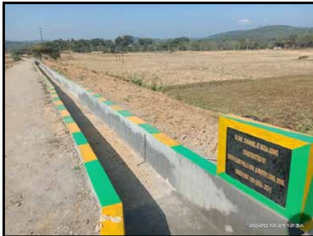
CC Irrigation Channel at Ruga Adinggre under RIDF XXV, South Garo Hills
