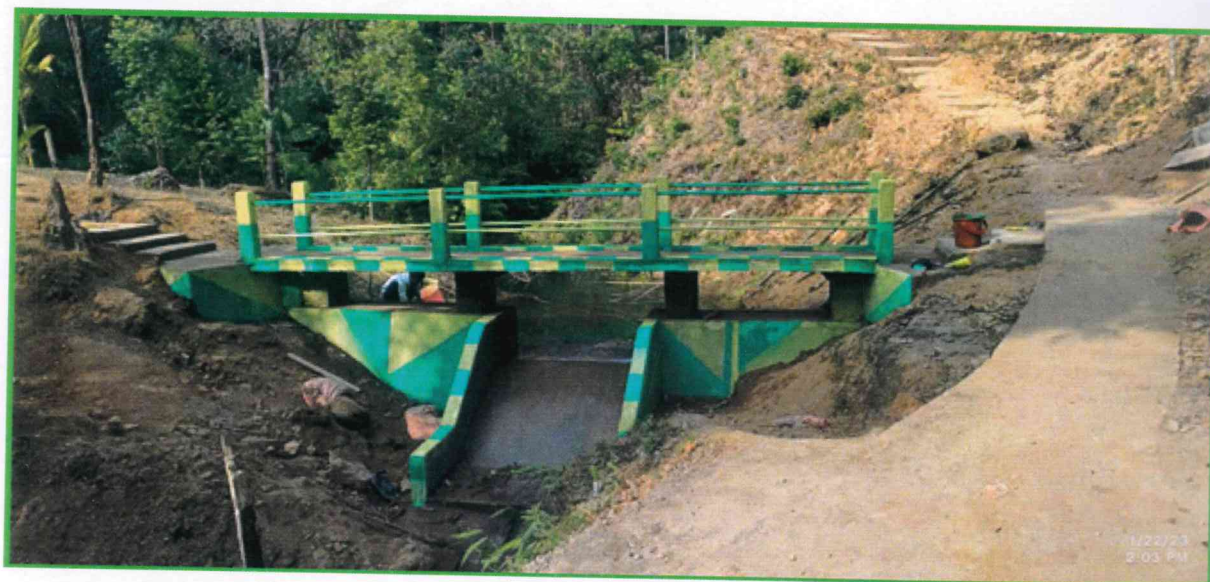
RCC Check Dam Cum Foot Bridge at Darang Dura South Garo Hills District
