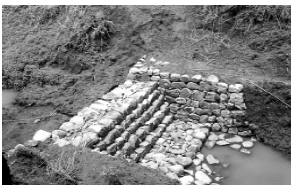
Gully control: strengthening the soil.
